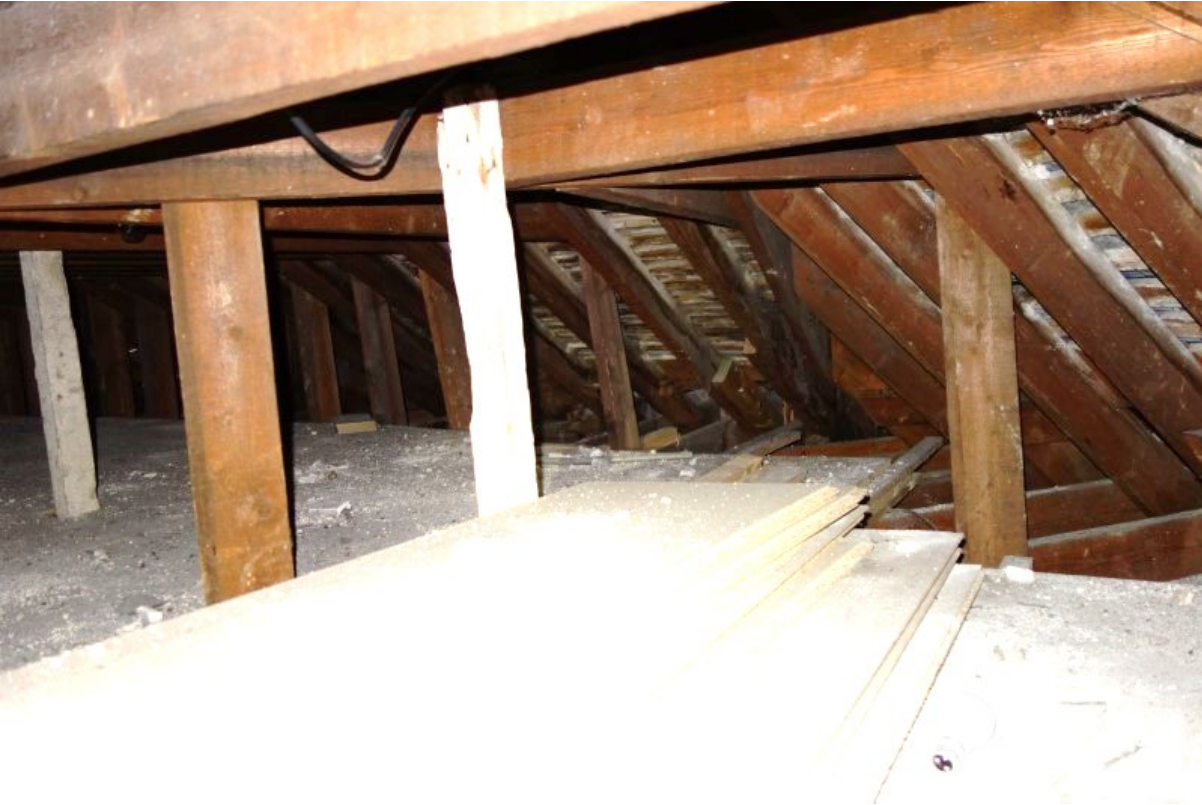
Figure 3: Interior of attic in original building
