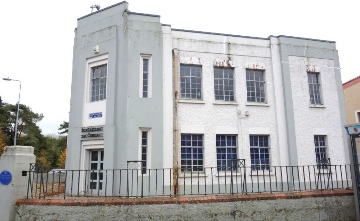
Figure 1: Exterior of original library building
