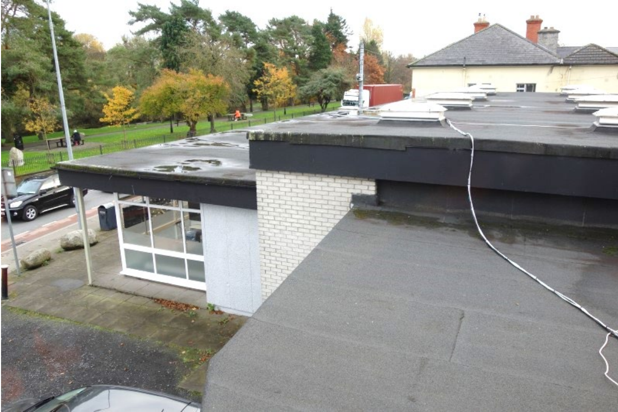
Figure 6: Flat roof of the single-storey building
